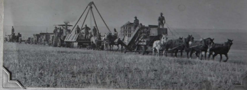
In the early days threshing crews moved from one ranch to another. This outfit consisted of threshing machine, derrick, steam engine, and water tank. A cook house was also in the outfit, which furnished meals for twenty men.
