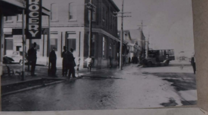
Water pouring down Main Street during thaw in February 1937. This picture was taken in front of Shannon's Grocery Store.
