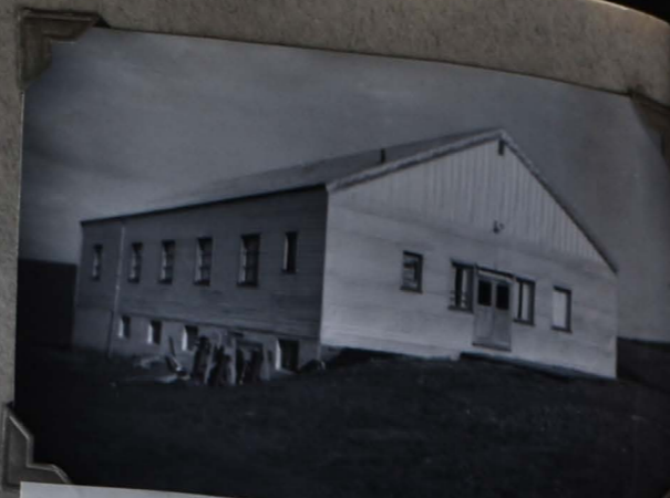
The new Igo Grange Hall completed in 1951, is located five miles west of Condon on highway 206.
