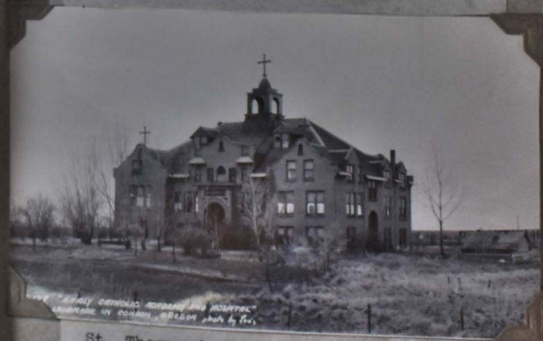
St. Thomas Academy and Hospital, built in 1909. The Catholic Church held its meetings here until 1925. This building has been vacant for many years.
