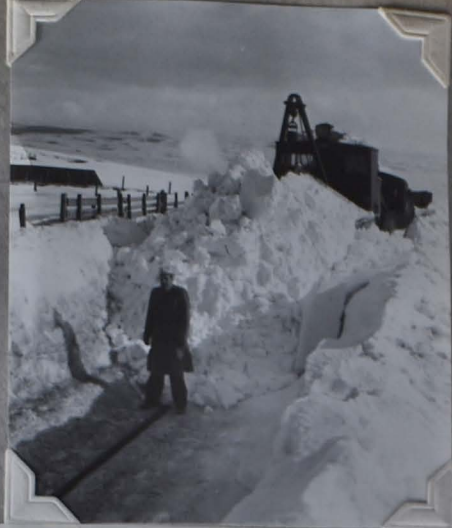
Snow plow clearing the Kinzua Railroad tracks. 1937
