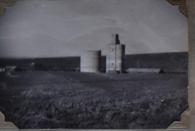
Concrete Grain Elevators at Mikkalo, completed in 1950.
