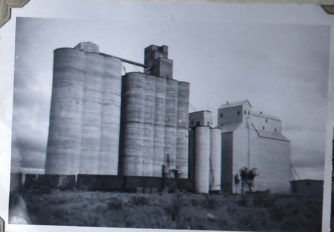
Three Grain elevators owned by the Condon Co-operative Grain Growers Assn. with a total storage capacity of one million Bu.
