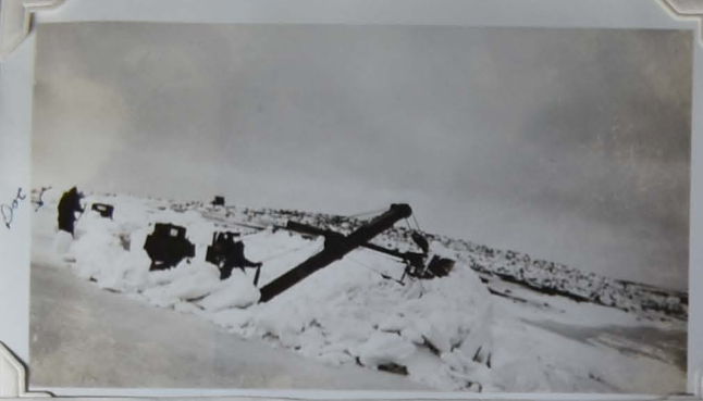
The snow was too deep for the snow plow. a steam shovel is being used to dig out the drifts.
