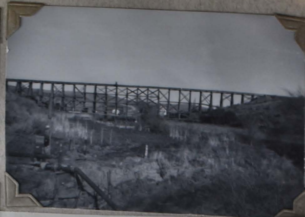
The Railroad bridge over Rock Creek at Rock Creek Station. Built in 1905 when the rail road came to Condon.
