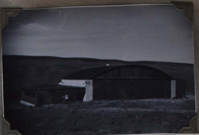
The Arlington High School Gymnasium. built in 1951.
