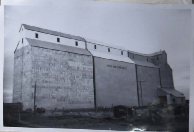
Elevator owned by Archer-Daniels-Midland Co. with storage capacity of 450,000 bu.
