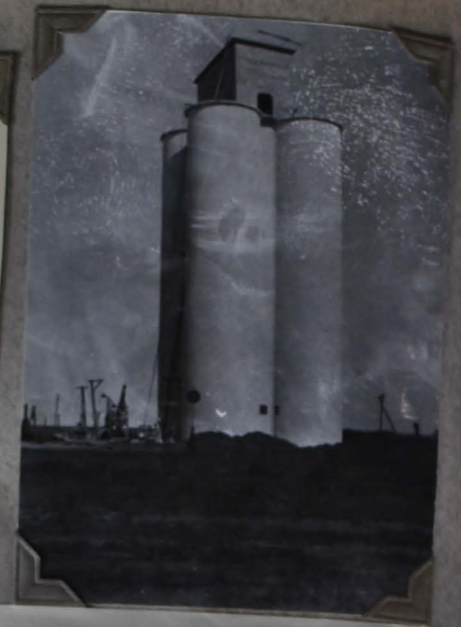
First Grain elevator in Condon built by the Farmers Elevator Co. in 1916. An annex was added in 1919, which was overloaded and collapsed in 1921.
