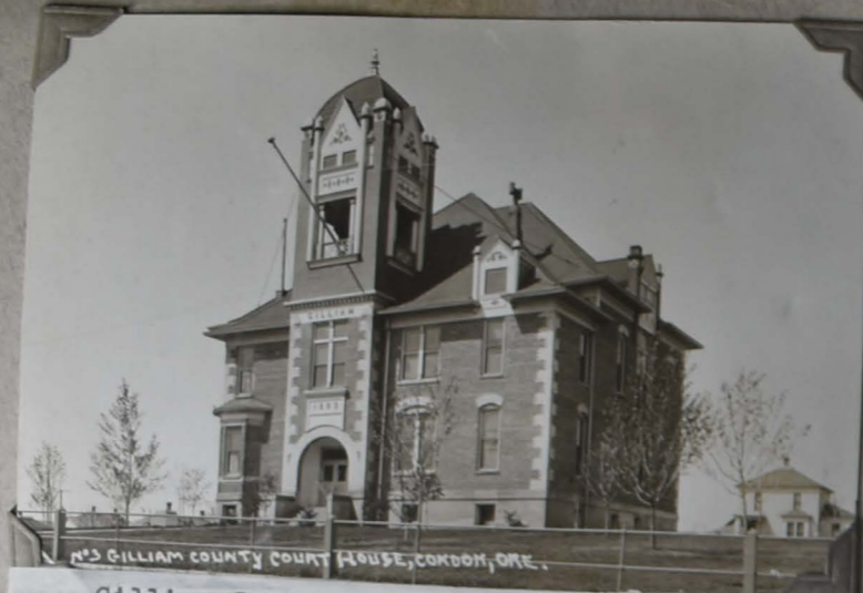
Gilliam County Court House built in 1903. At a cost of $17,000. The material was furnished from the local brick yards. The first officers to occupy this building were T. G. Johnson, Sheriff, and C. O. Portwood, Treas.
