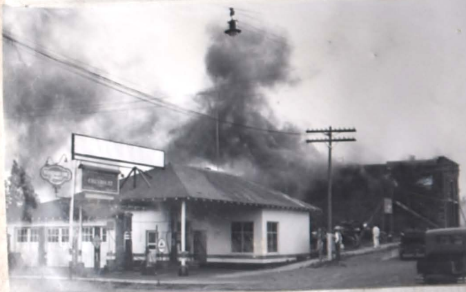
In Aug. 1932 fire destroyed the Kingsley Blacksmith Shop and the Harrison Stone building. Smoke can be seen pouring from the building.
