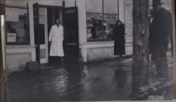
When the snow melted in Feb. 1937, the water came through Brandt's Meat Market. Dick Brandt in doorway, Nell Brandt by window, and Jim Ramsay by Light pole.
